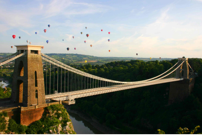
Figure 9.1: Clifton suspension bridge, Bristol, UK. The cables of a suspension bridges hang in a shape which is almost (but not exactly) a parabola.
