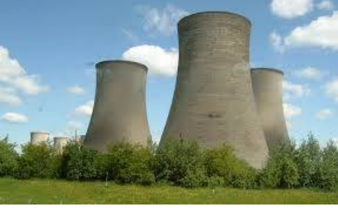
Figure 9.9: Cooling towers. Şekil 9.9:
