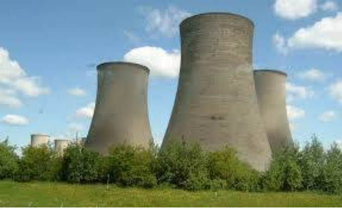
Figure 24.9: Cooling towers. Şekil 24.9:
